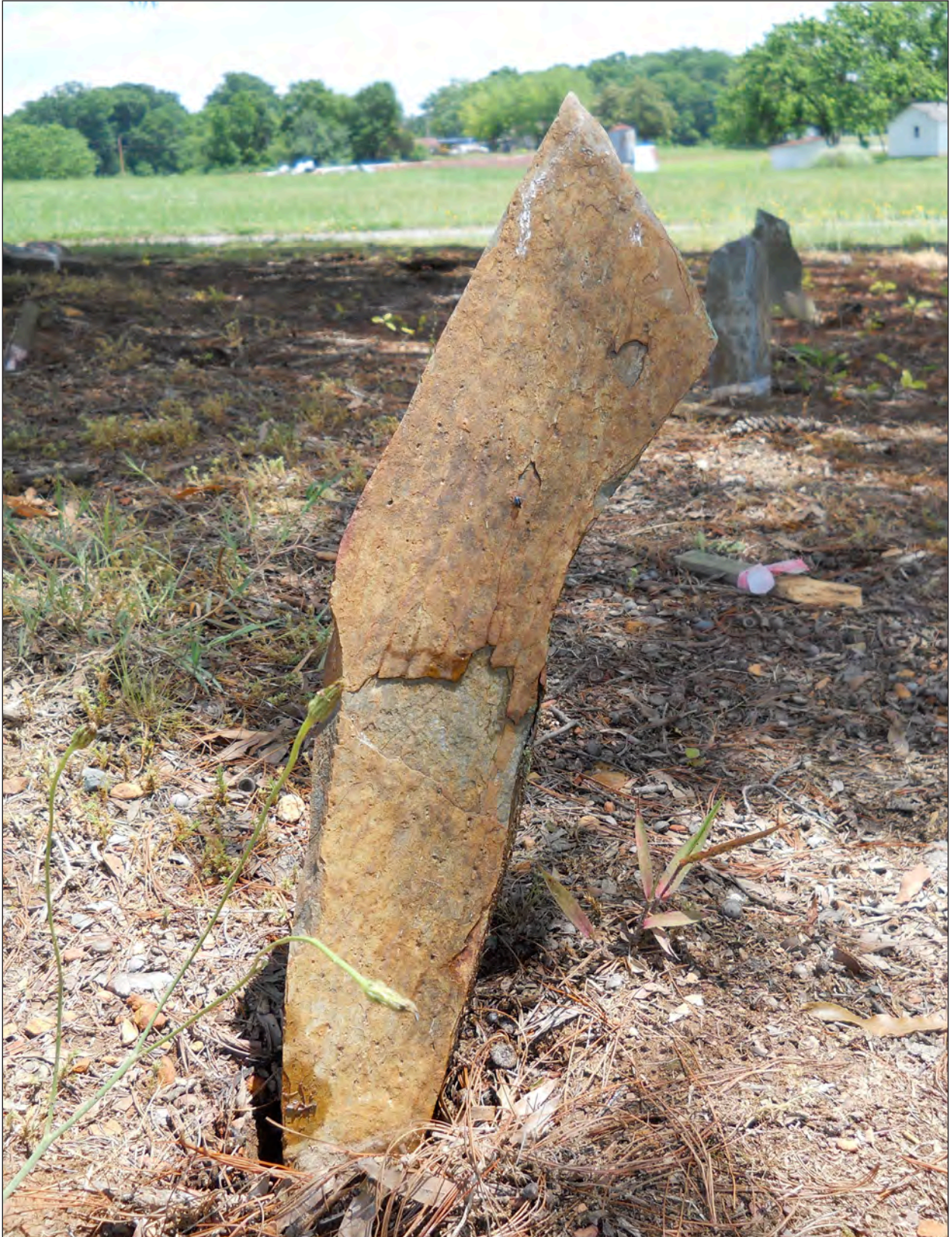
Figure 9. Photograph of Marker Number 3, Loose and Leaning
