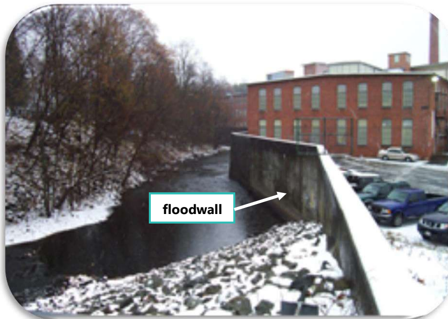
Figure 3.3 – Example Floodwall – Framingham, Massachusetts
