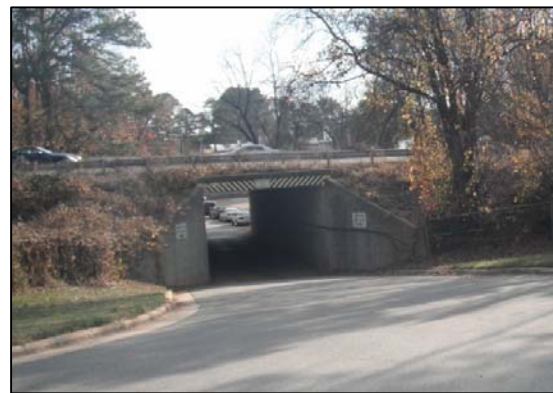
Ligon Street one-lane tunnel under I-440
