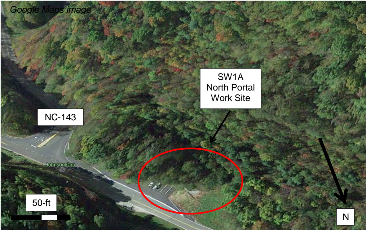
Figure 6: Aerial image from Google Maps showing the north portal worksites for alignments S2 and SW1A
