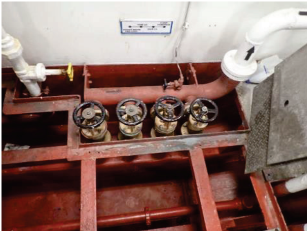
Reworked/new valve on vessel in shipyard
