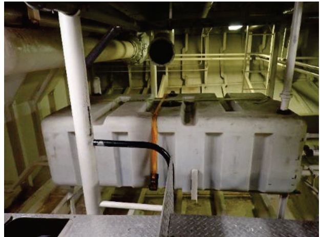
Sewage holding tanks installed on older vessel for operation in no discharge zone (Southport to Fort Fisher)
