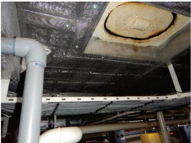
Neat cable way on newer vessel
