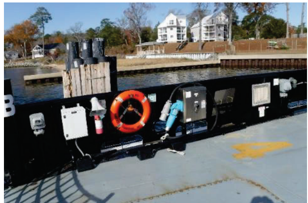
New vessel fire extinguisher and ring buoy typical for all vessels
