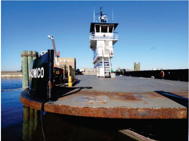
Deck and hull condition of older Hatteras class vessel
