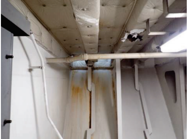
Interior structure in way of outside vent
