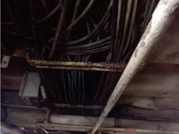
Wiring arrangement of older vessel note blackened cables
