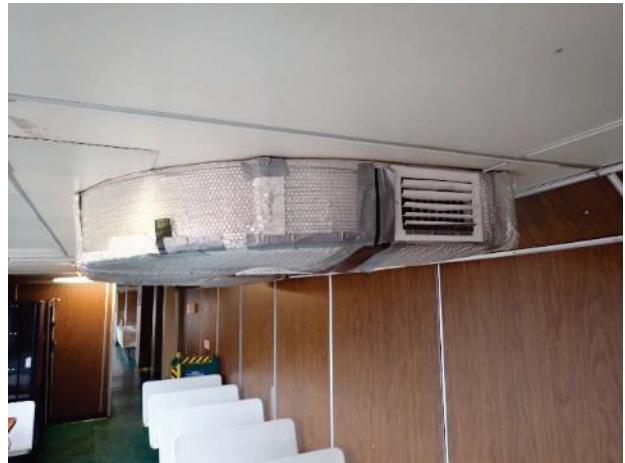
Duct system for non mini split system
