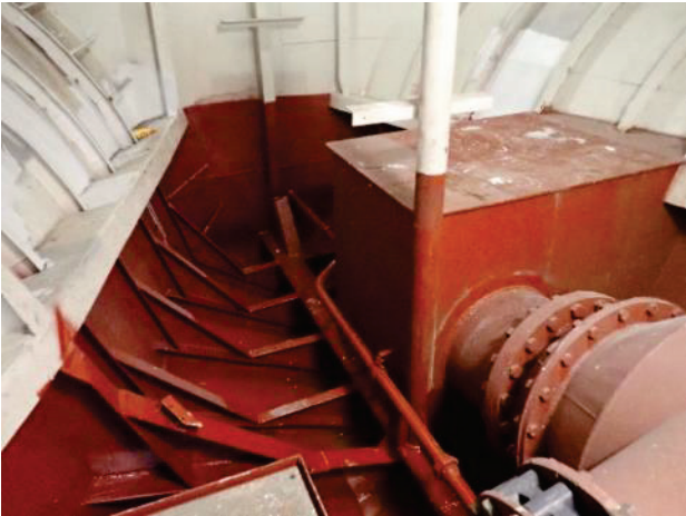
Typical sea chest and piping on older vessel in bilge area
