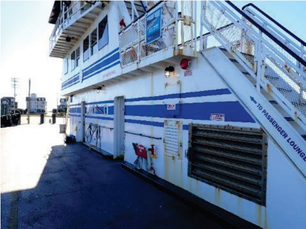
Structure view showing corrosion
