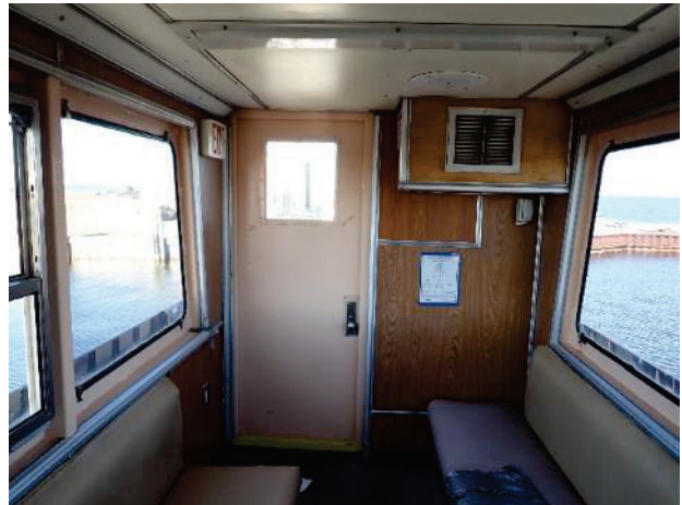
HVAC duct on older vessel
