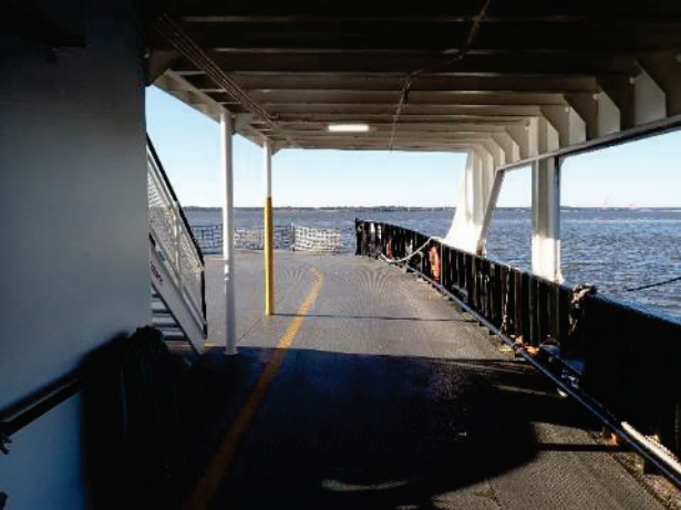
Typical car deck and lane of passenger ferry
