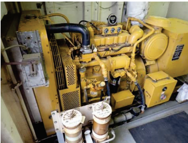
Non-tier older generator and engine
