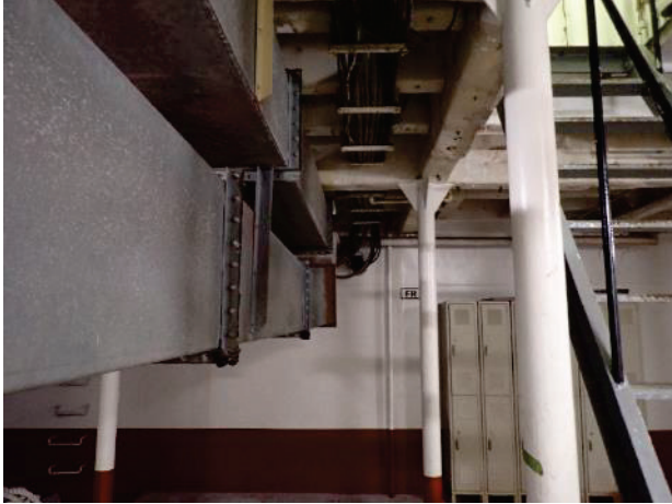
Typical ducting for central HVAC
