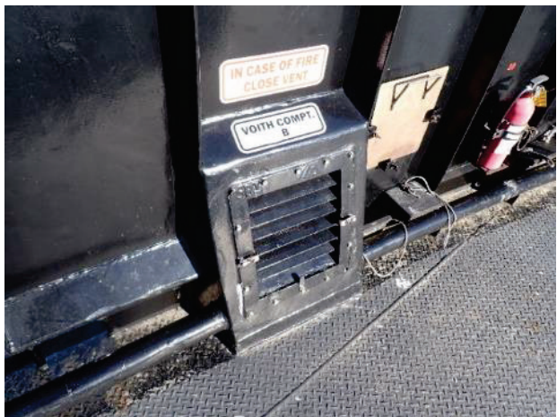
Compartment vent with blanking plate
