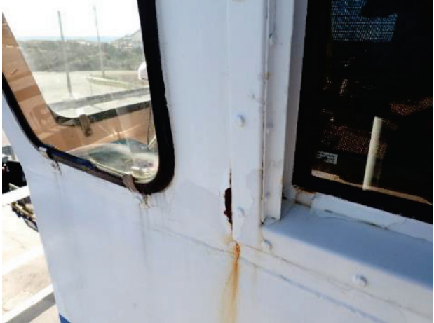
Typical condition around windows as vessels age
