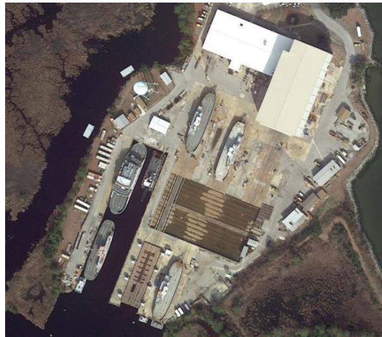
FIGURE 4.2 Aerial View of Manns Harbor Maintenance Facility
