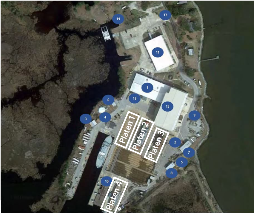
FIGURE 2.2 Aerial View of Manns Harbor Maintenance Facility
