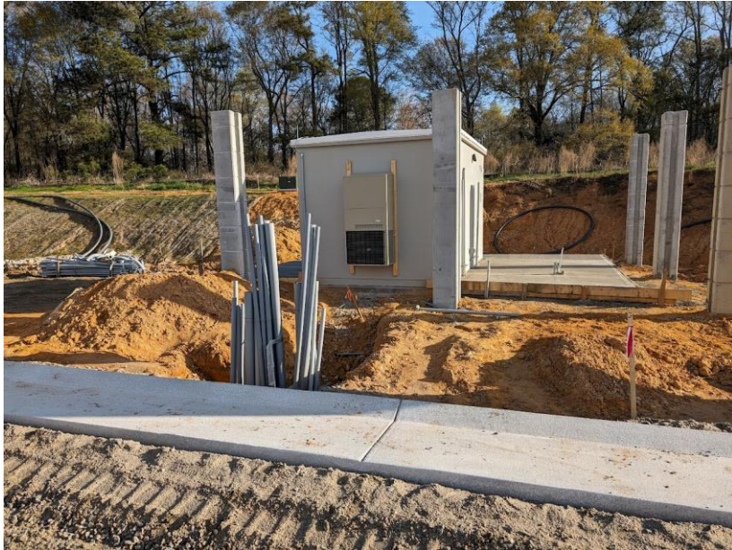
Contractor crews installing vault building at Site 4 on R-2828
