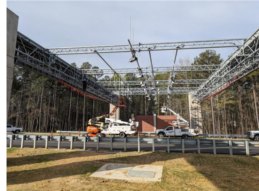
Kapsch crews installing overhead toll equipment at Site 3 on R-2721B
