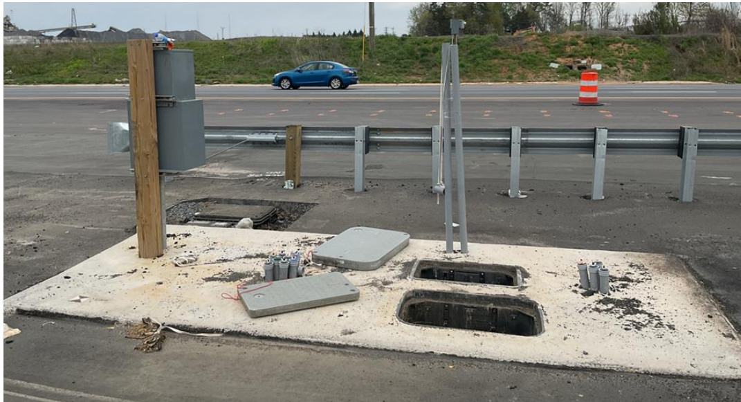
Conduit and Pull Boxes Installed, Concrete Pad Poured
