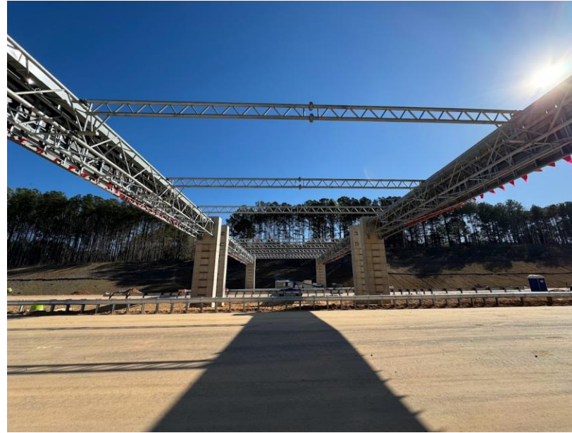
Toll Site 1 ready for turnover on R-2721A
