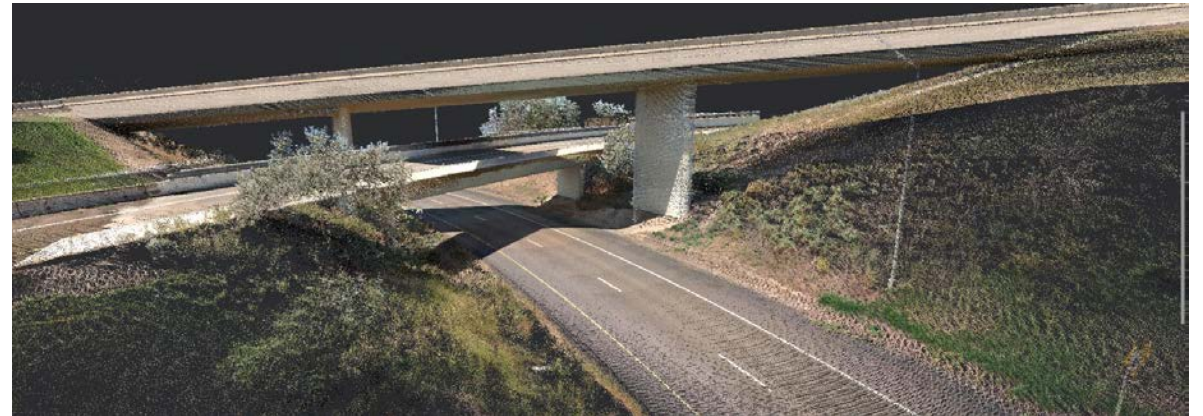
LiDAR imagery courtesy of CycloMedia.
