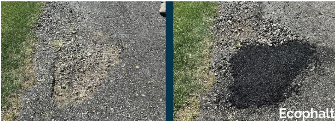
Image of a repaired pothole using Ecophalt™.
