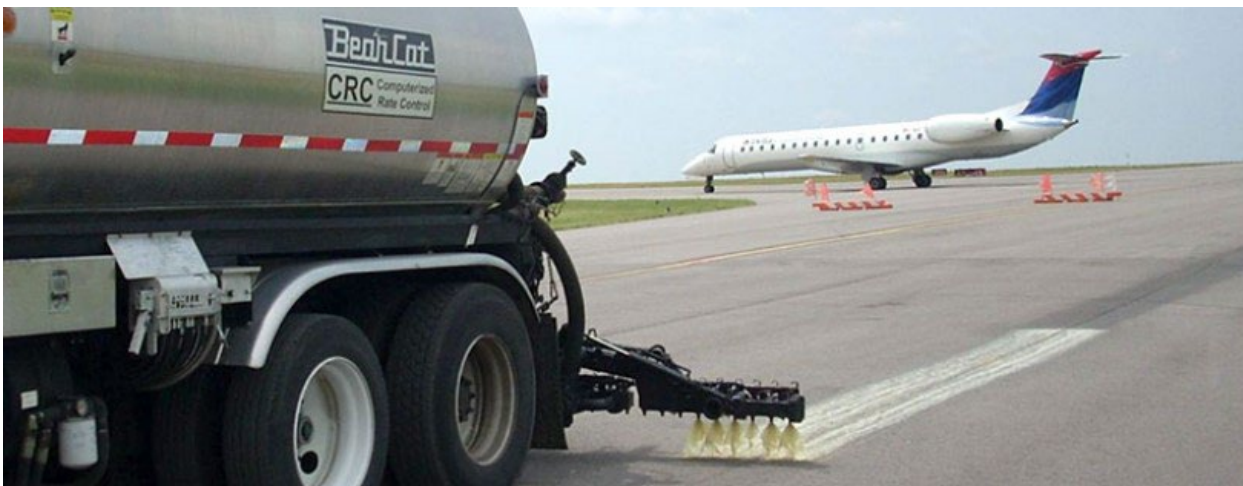
Image of JOINTBOND® being applied from Pavement Technology's website.
