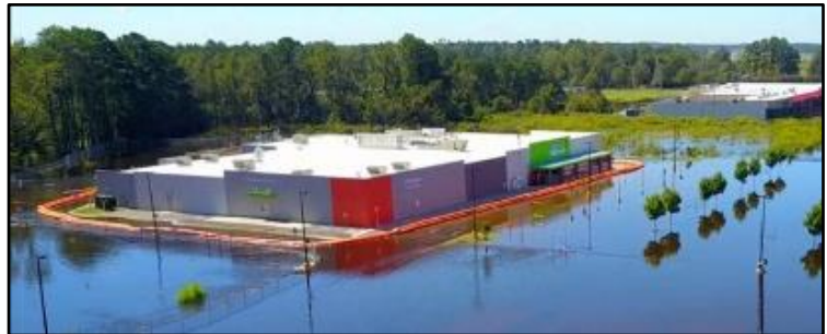
Tiger Dam™ protecting a Wal-Mart in North Carolina during a flood event – image from U.S. Flood Control Website
