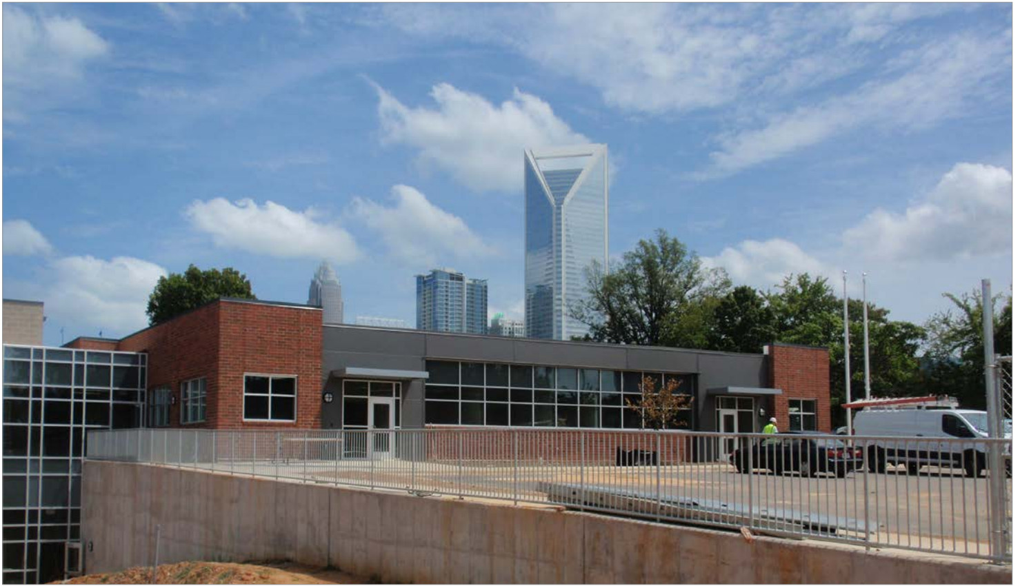
Front entrance of Charlotte Locomotive and Railcar Maintenance Facility office building
