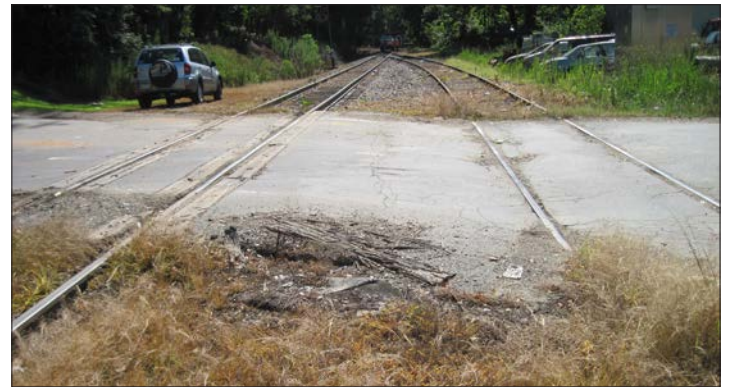
Mineral Springs Road before improvements
