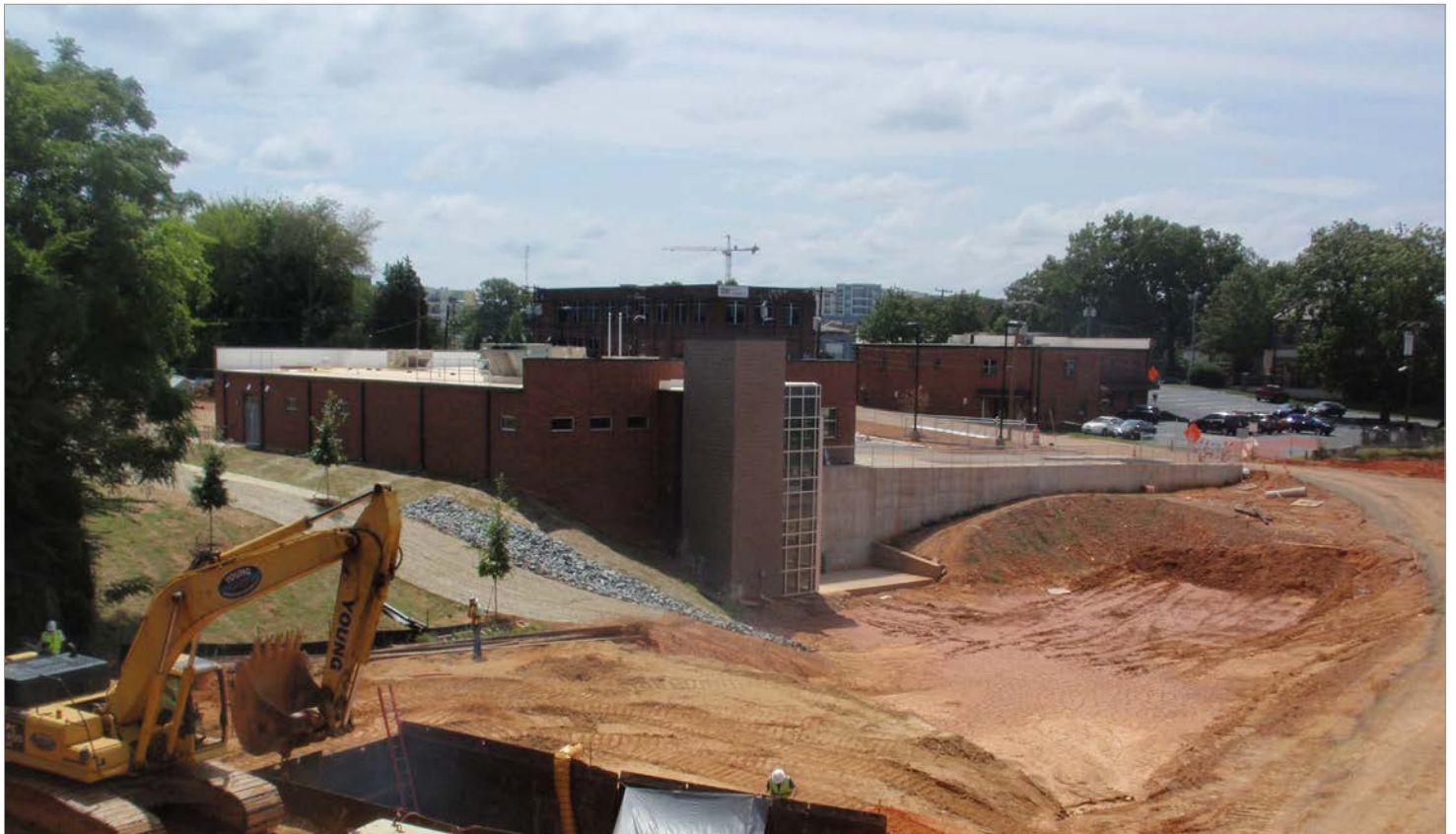
Grading work at rail yard side of office building
