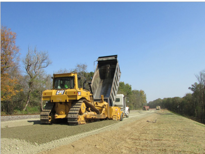
P-5208 Haydock to Junker, sub-ballast
