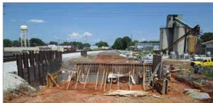
Klumac under construction, June 2014
