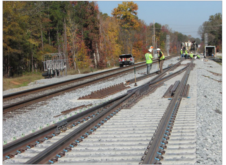
P-5206 Reid to North Kannapolis, track construction
