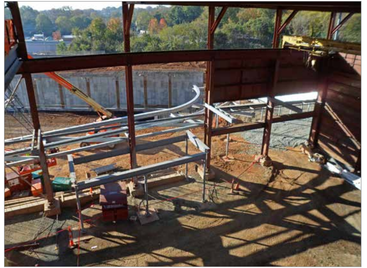
P-5500 Raleigh Union Station construction
