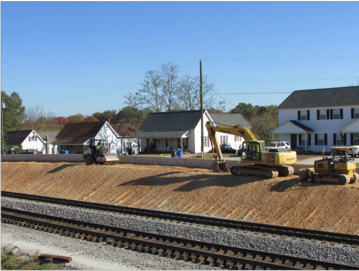
P-5206 Reid to North Kannapolis, track construction
