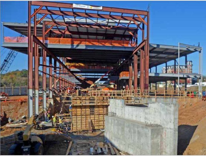
P-5500 Raleigh Union Station construction
