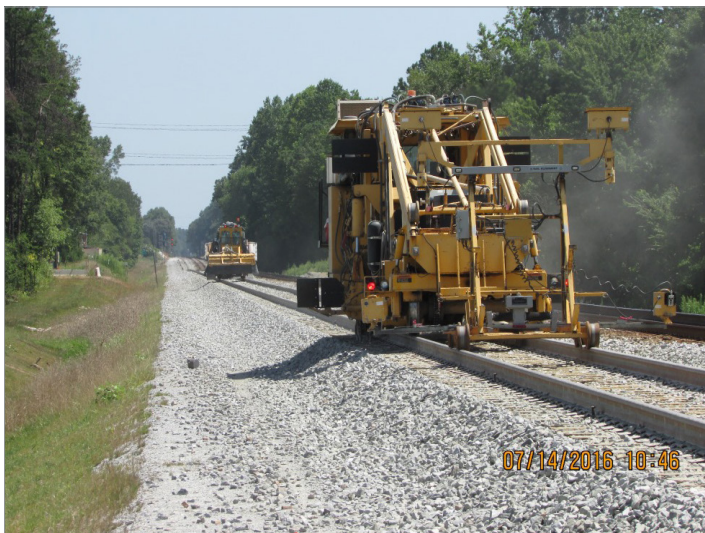
P-5206 Reid to North Kannapolis, track construction
