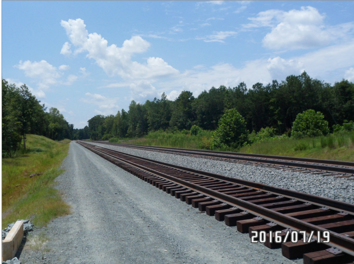
P-5205 Graham to Haw River Passing Siding, siding track construction
