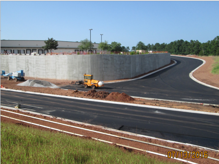
P-5201 Morrisville Parkway, retaining wall
