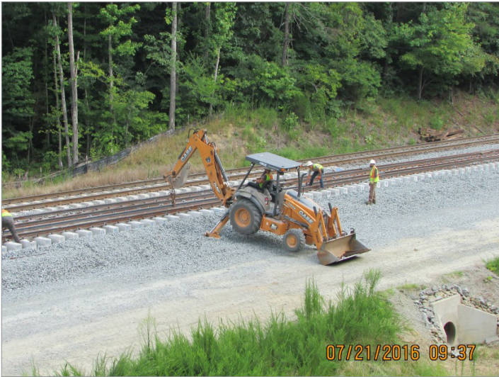
C-4901 Bowers to Lake, track construction
