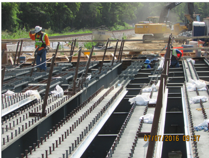
P-5208 Haydock to Junker, Coddle Creek, bridge construction
