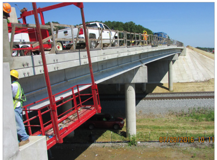
P-5208 Haydock to Junker, Roberta Road bridge construction
