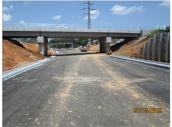
U-3459 Klumac Road, roadway paving
