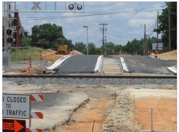
P-5206 Reid to North Kannapolis, 22nd Street roadway construction
