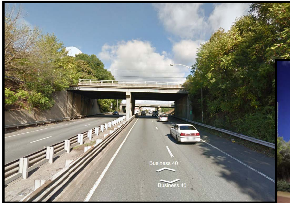
Marshall Street Bridge
