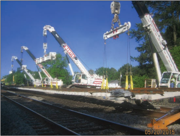
P-60 Congestion Mitigation – Enfield Turnout Construction
