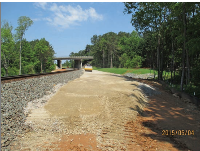
P-5500C Tryon Siding grading
