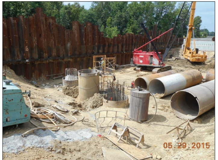
P-5208 Haydock to Junker, bridge column construction
