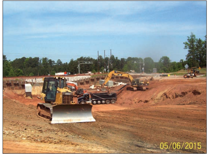
P-5201 Morrisville Parkway, grading
