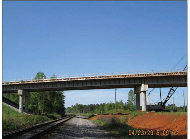
P-5206 Peeler Road, bridge construction
