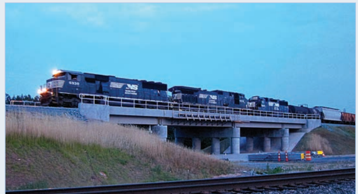
First train crossing new railroad bridge over Hopson Road.
