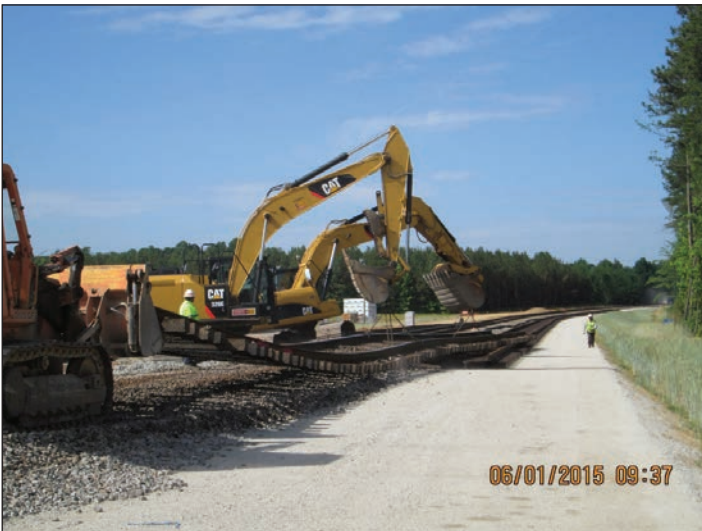
P-5206 Reid to North Kannapolis, track construction
