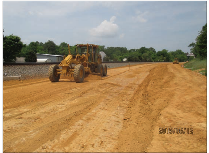
P-5205 Graham to Haw River Passing Siding, grading
