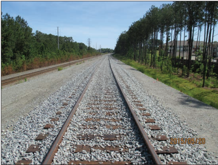
U-4716 Nelson to Clegg Passing Siding, track construction
