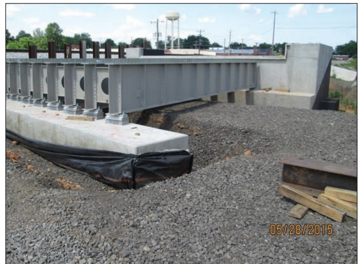
U-3459 Klumac Road, bridge construction
