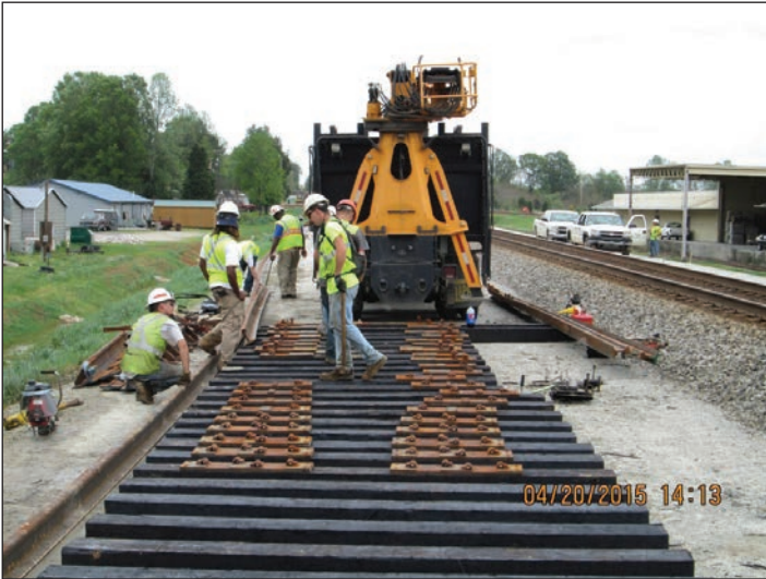
P-5206 Reid to North Kannapolis, track construction
