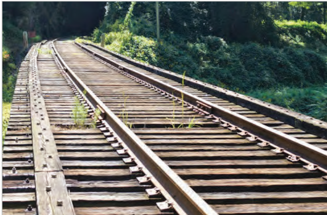
Great Smoky Mountain Railroad bridge
