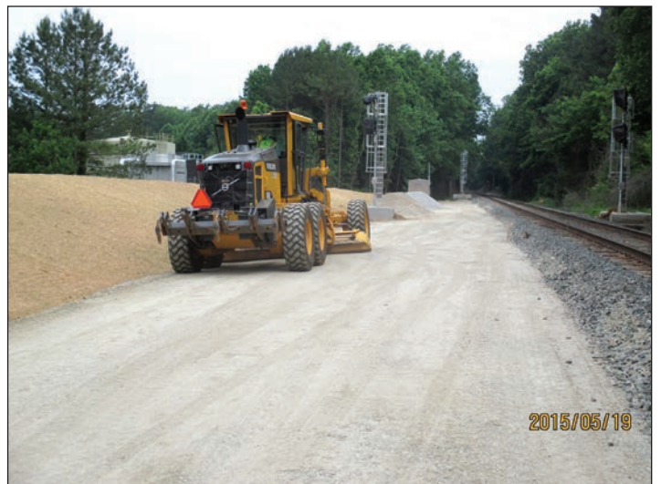
P-5500C Tryon Siding sub-ballast
