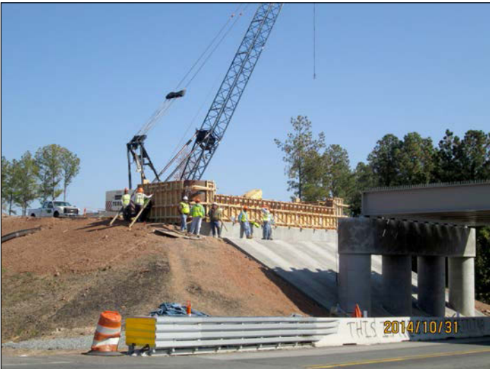
U-4716 Hopson Road bridge construction
