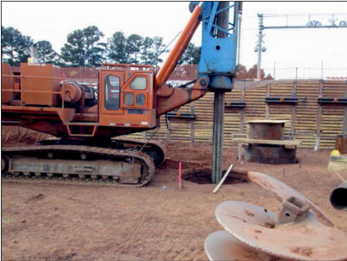
P-5201 Morrisville Parkway, west approach to bridge
