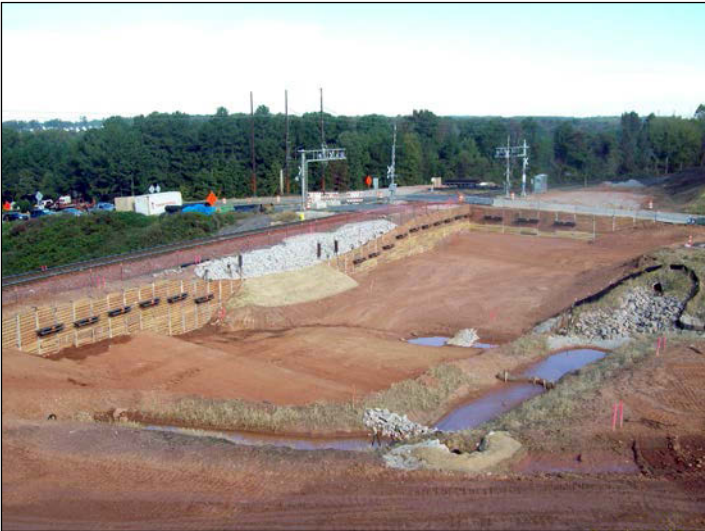
P-5201 Morrisville Parkway grading
