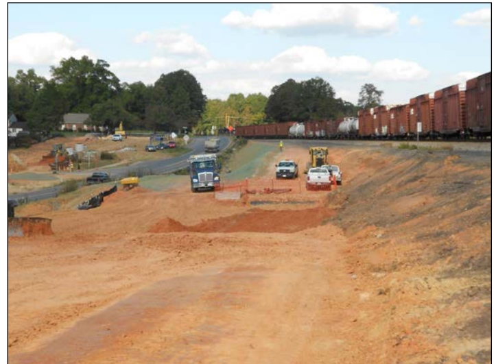
P-5208 Haydock to Junker - Grading
