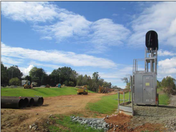
P-5205 Graham to Haw River Grading
