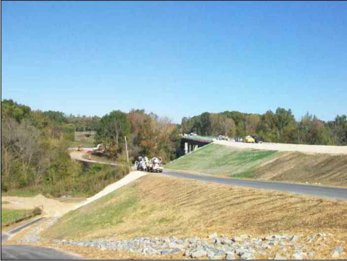
C-4901 Bowers to Lake - Turner Road Bridge Paving
