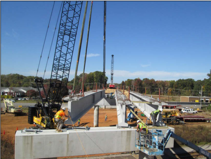
P-5206 Reid to N. Kannapolis - Peeler Road Bridge Construction
