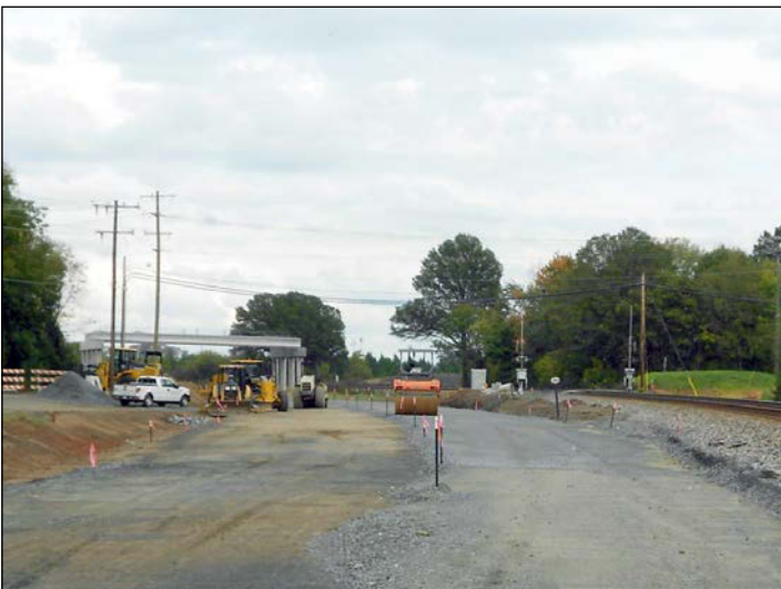
P-5208 Haydock to Junker - Roberta Road Bridge
