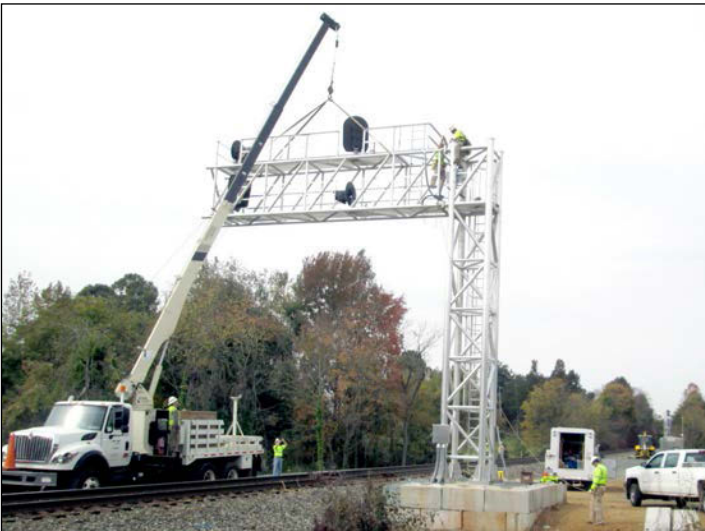
P-5205 Graham to Haw River, signal installation
