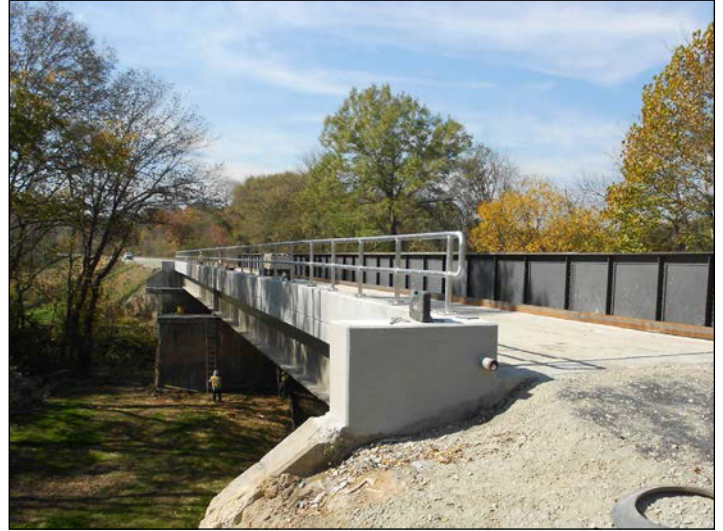
C-4901 Bowers to Lake - Bridge over Abbots Creek
