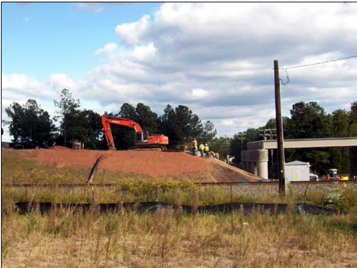
U-4716 Hopson Road bridge construction
