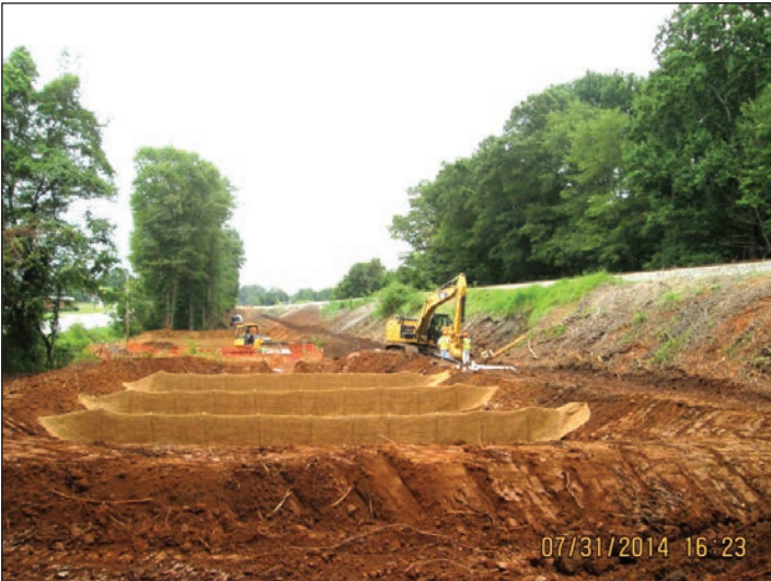
P-5206 Reid to N. Kannapolis - Erosion Control
