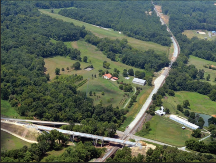
C-4901 Bowers to Lake - Turner Road Bridge
