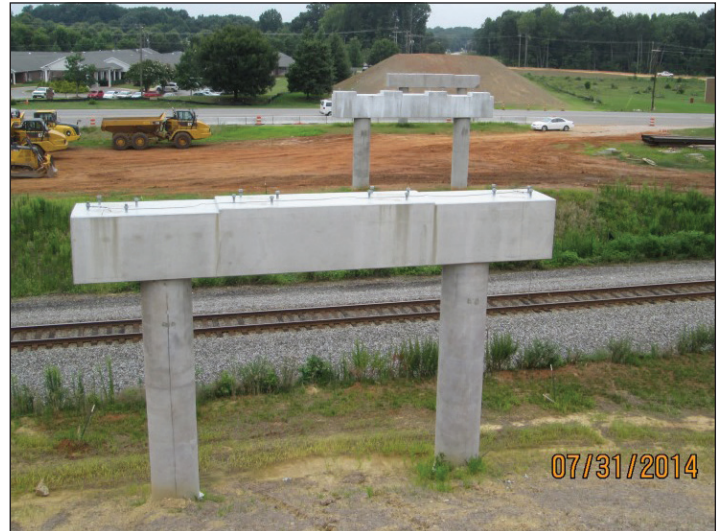
P-5206 Peeler Road Bridge Construction
