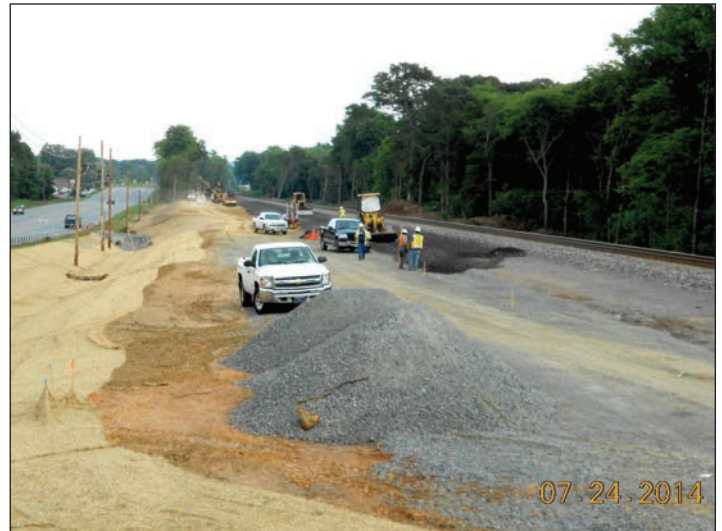
P-5208 Haydock to Junker - grading
