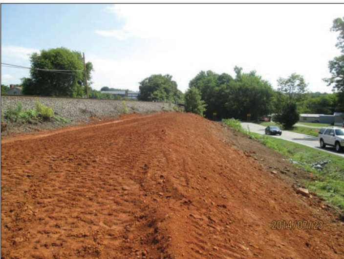
P-5205 Graham to Haw River Grading
