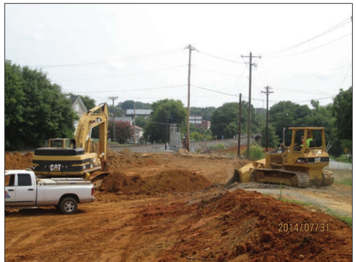
P-5205 Graham to Haw River Grading
