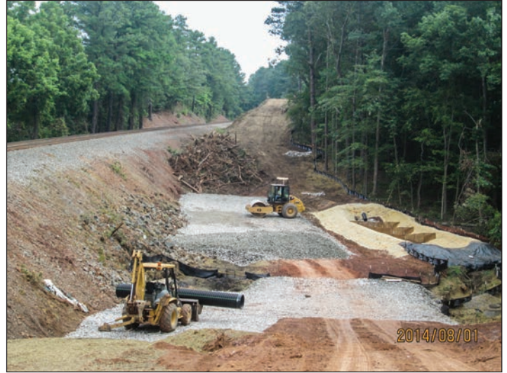
P-5201 Morrisville Parkway, west approach to bridge
